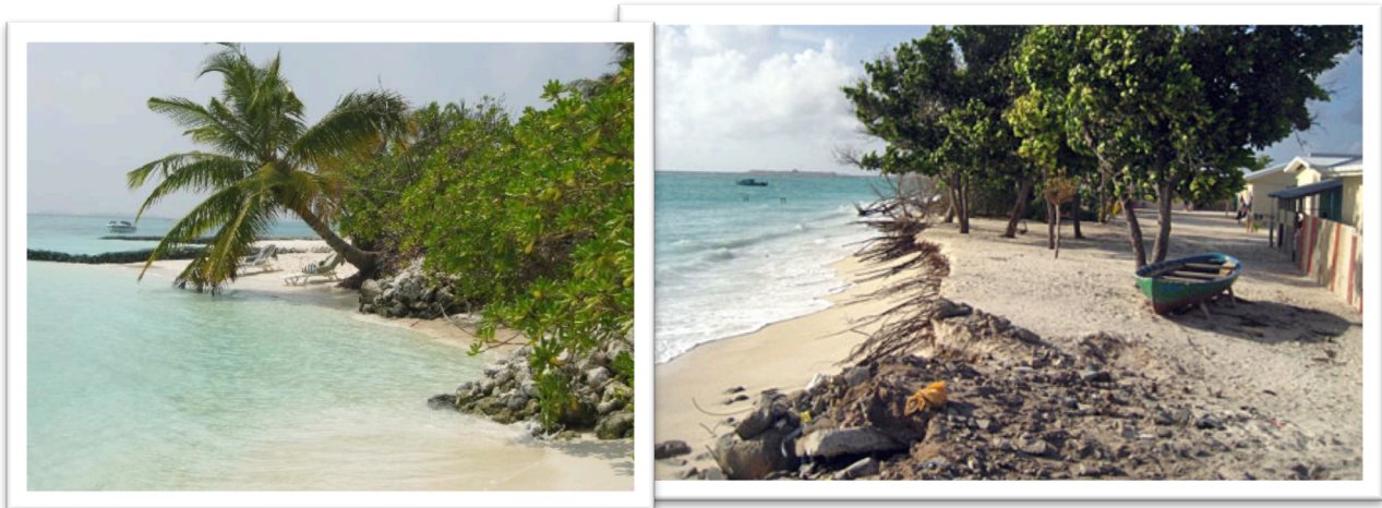
Erosion in the islands
